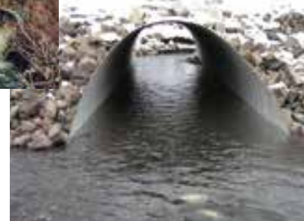
Culverts (above left) prevented fish from freely moving from Maggie Creek into Beaver Creek, a major tributary. In 2005 they were replaced with this fish-friendly structure (above) to connect the streams.
