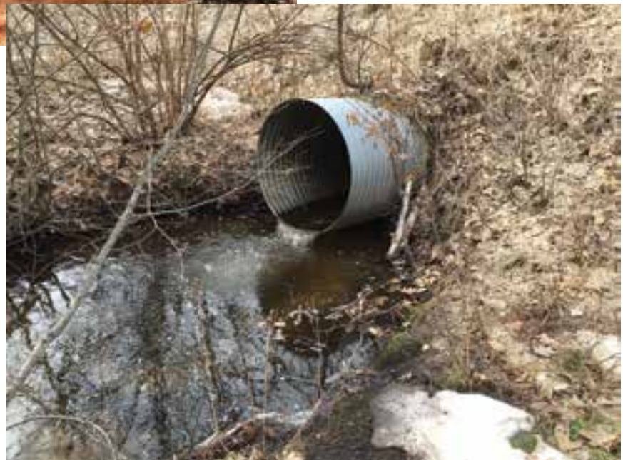
Perched culvert in Northern MI.
