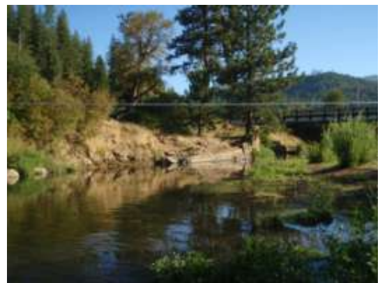
X-Sec 1 2011, looking downstream
