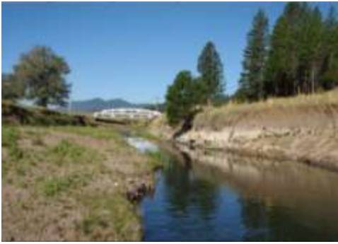
X-Sec 1 looking downstream
