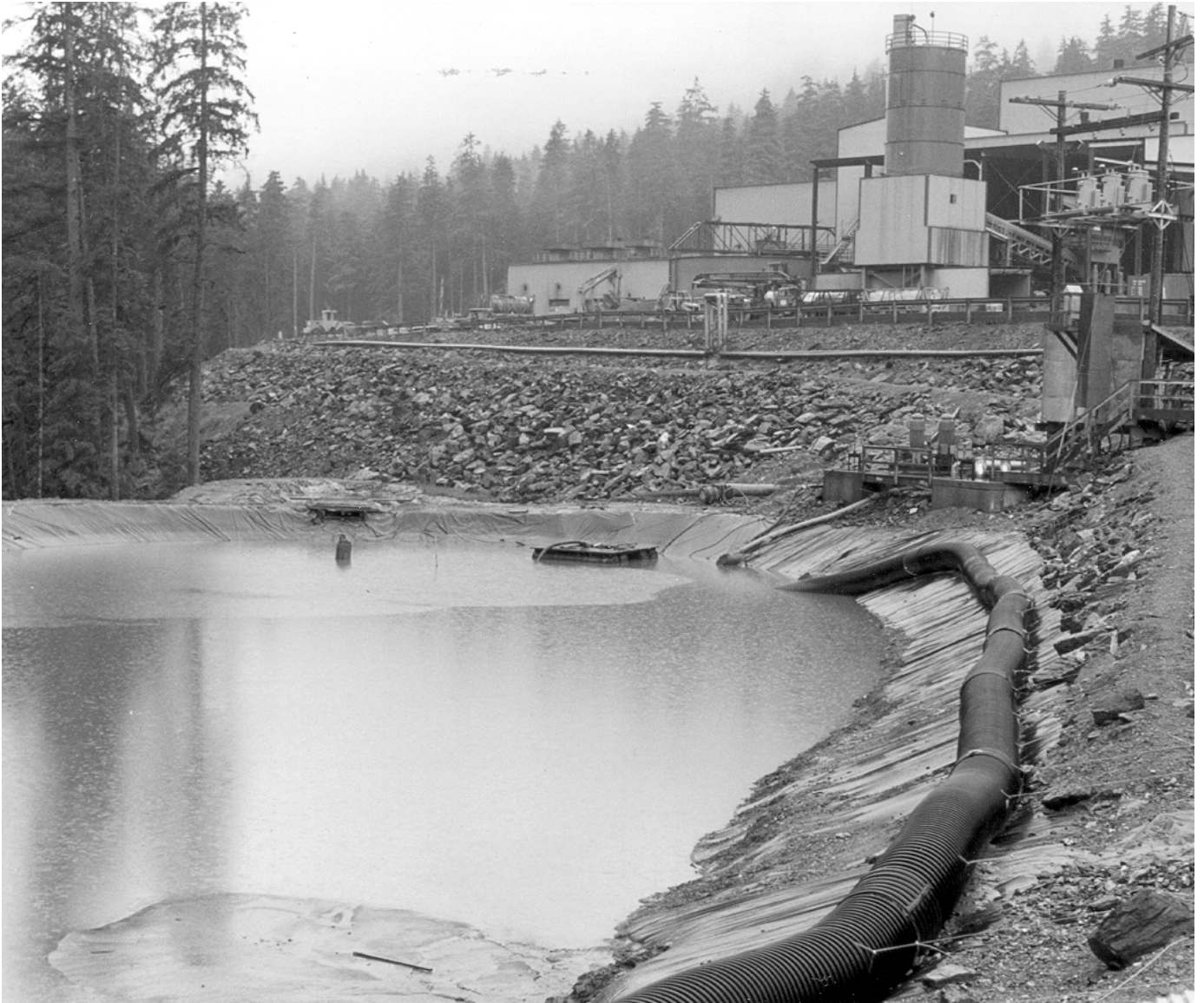
Greens Creek Mine, Tongass National Forest, Alaska, with sediment pond. Photo by Stephen Glasser
