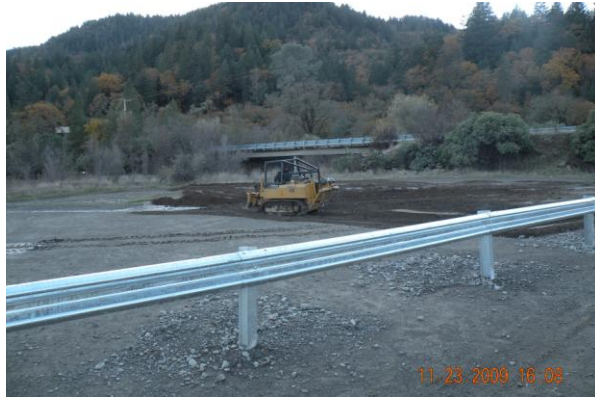
Photo 1 (Before): Picture is taken looking toward the Elk Mountain Rd bridge over the West Fork of Middle Creek. In the foreground is the OHV riding area being subsoiled to alleviate compaction. The highly compacted riding area would contribute significant amounts of runoff and fine sediment into the West Fork during even frequent low-intensity rainfall events.
