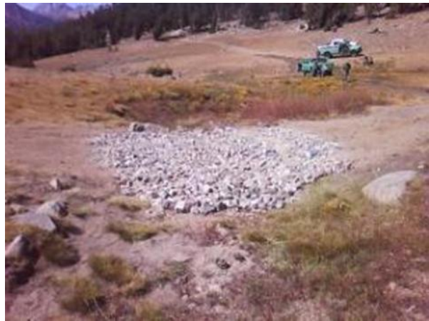
Drainage hardening at seasonal stream crossing to prevent erosion and further headcutting on Trail #31E301.
