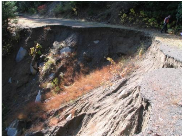
Pre-project photo of fill failure on road 40N51
