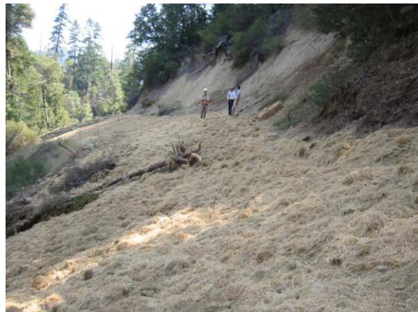
Fill removed from the stream crossings as well as recontouring the swales results in a gently outsloped road as part of the final road decommissioning work.
