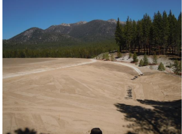
Photo 4: The last steps of the Meyers landfill restoration prepare the surface soils for seeding.
