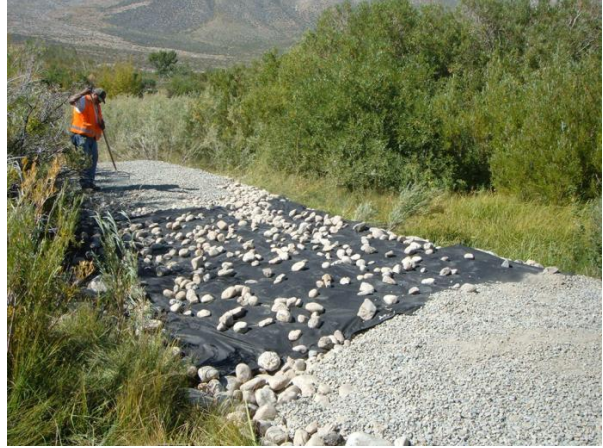
Project near completion with an extra layer of cobble on top of the crush to facilitate proper drainage.
