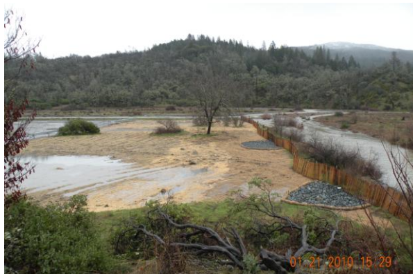
Photo 2 (During): Picture was taken from the bridge over West Fork Middle Creek the first winter after completion. Straw was used to stabilize the area until vegetation could take hold. Overland flow can be seen ponding in depressions allowing the majority of the runoff to infiltrate back into the soil and deposit fine sediments instead of spilling into West Fork. Also seen in this picture are two of the rocked outlets that were constructed for infrequent high-flow events. Rocked and waddled outlets also helped trap sediment. These outlets serve to also direct return flow back into the West Fork when it floods over its banks into the area.
