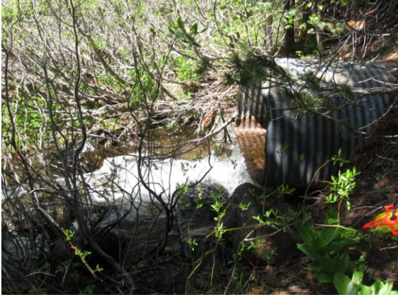
Culvert at the Pine Creek crossing of Road 25N29 on the Mount Hough Ranger District. Left photo shows the crossing prior to restoration, with a significant drop to the creek impairing passage for fish and other aquatic organisms. Right photo shows the crossing after restoration with streambed substrate and retention weirs.
