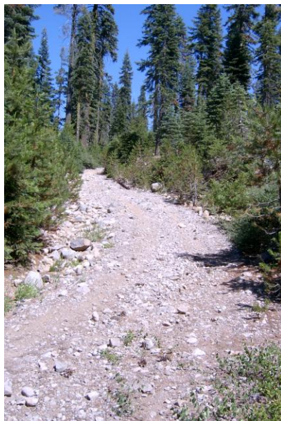
Before Road intact
