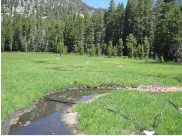
Photo 6: Irrigating the new channel for the North Fork of Cold Creek to help fully re-establish meadow vegetation.
