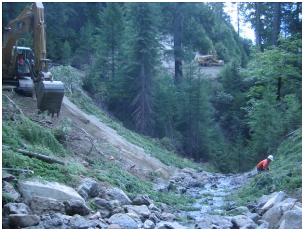
Photo of perennial stream crossing being decommissioned. Karuk Tribal members are operating the equipment and placing the final erosion control on the side slopes.
