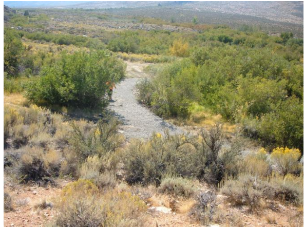
Completed rock causeway project to protect water quality, riparian resource and provide for a sustainable driving surface.
