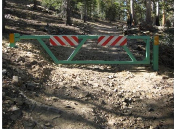
Finished seasonal gate on Road # 02N135. The closed gate will prevent wet weather traffic on the road, minimizing rutting and potential off-road erosion and stream sedimentation.
