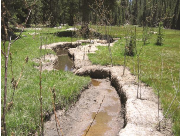
Loggy Meadow Restoration Project on the Sequoia National Forest. The project stabilized stream banks and allowed the stream to access its flood plain, returning the area to a more natural condition.
