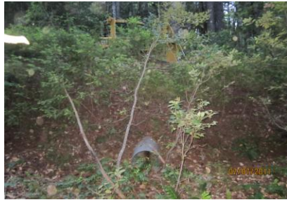
View of culvert and fill prior to being decommissioned.
