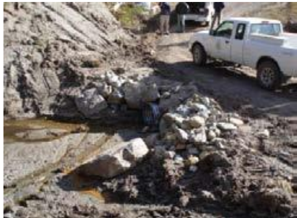
Post-project photo of Kanaka Creek crossing
