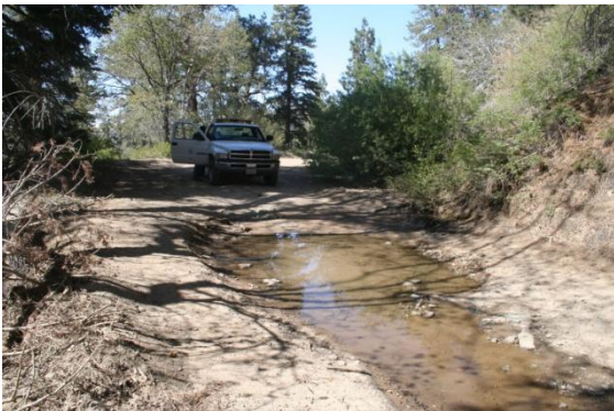
Before: Spring drains down road.
