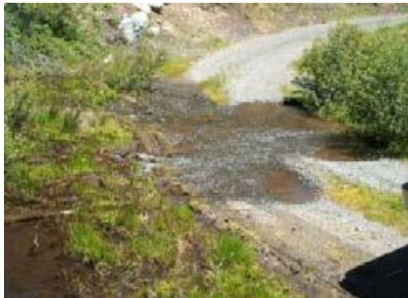
Pre-project photo of Kanaka Creek flowing over road
