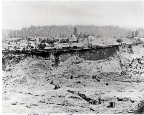
Hydraulic diggings near Camptonville, one of the local communities near the forest boundary and site of the Yuba River Ranger Station. From the collection of Leland Pauly.
