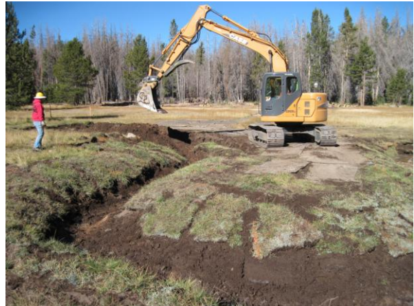
Photo 5: Cutting a new stream channel for Cold Creek in High Meadows.
