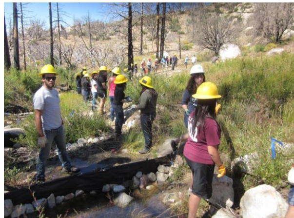
Paramount High School Environmental Club assists with meadow repairs.
