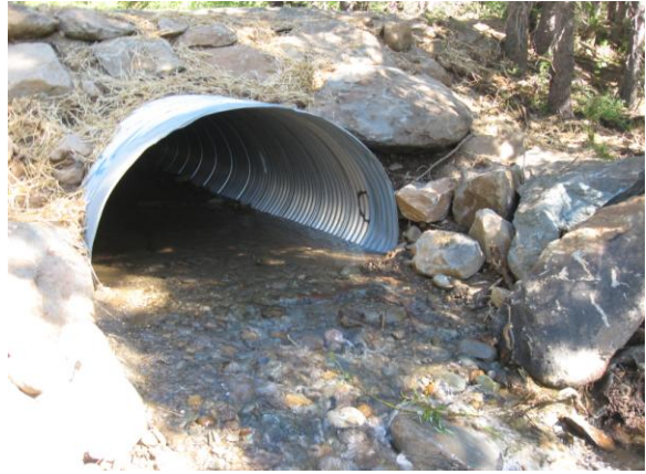
Culvert at the Pine Creek crossing of Road 25N29 on the Mount Hough Ranger District. Left photo shows the crossing prior to restoration, with a significant drop to the creek impairing passage for fish and other aquatic organisms. Right photo shows the crossing after restoration with streambed substrate and retention weirs.
