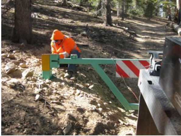
Putting the final touches on a seasonal closure gate near the Boy Scout Mine on the Mono Lake District (Road #02N135 ).
