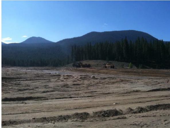
Photo 4: The last steps of the Meyers landfill restoration prepare the surface soils for seeding.
