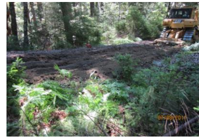
This photo shows how the dozer uses the rippers to decompact the road surface. This technique promotes infiltration and new vegetation growth. Native grass seed is spread to provide cover until other shrubs and trees become established.
