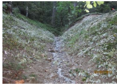
View looking upstream of newly constructed perennial stream crossing.
