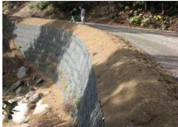
Post-project photo of retaining wall
