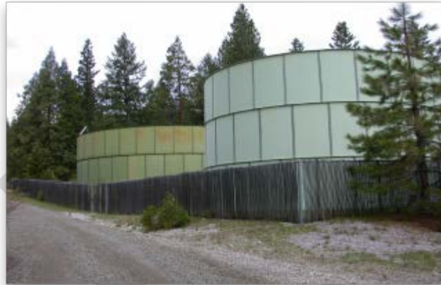
Water tanks (Source: Plumas-Eureka CSD)
