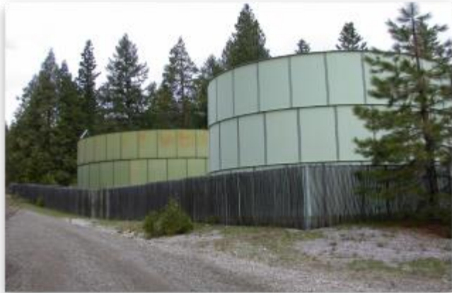
Water tanks (Source: Plumas-Eureka CSD)
