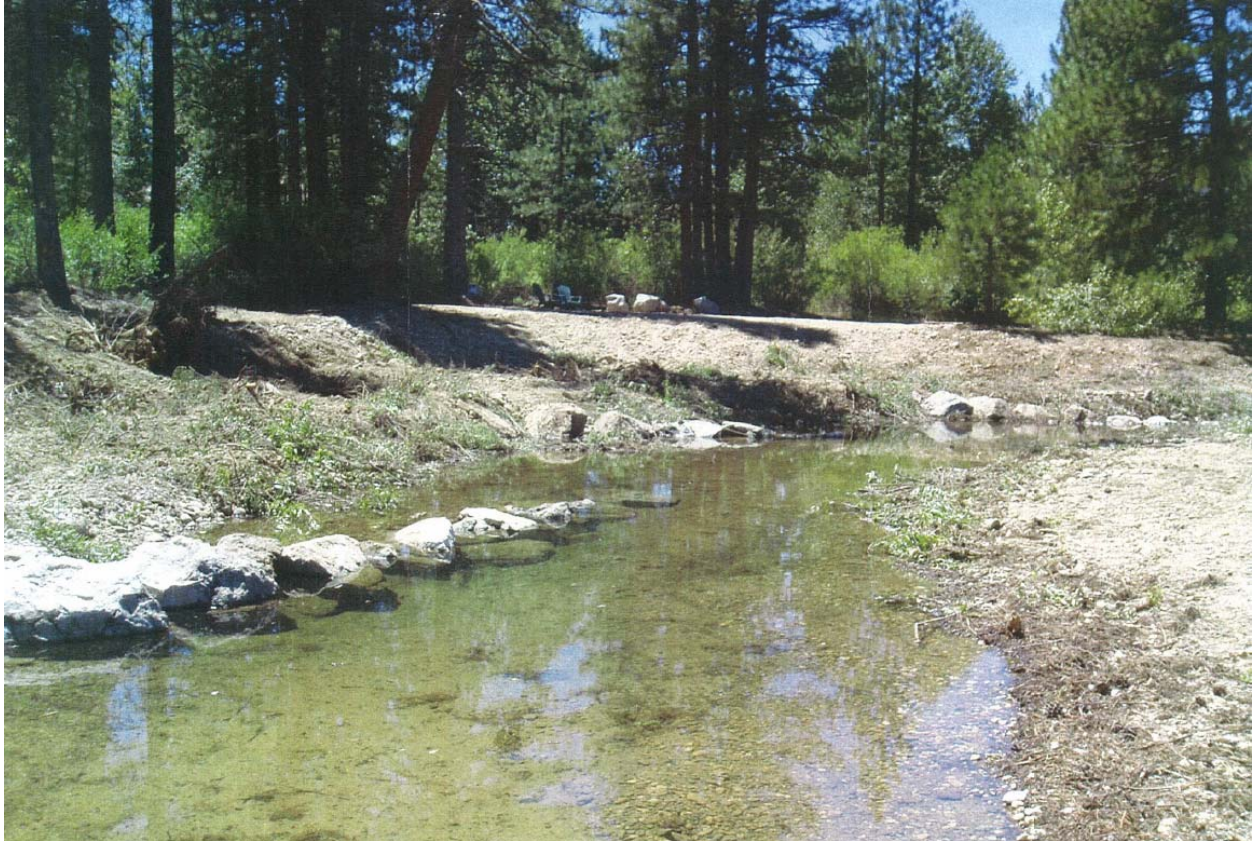
Boulder Vanes Constructed on Spanish Creek
