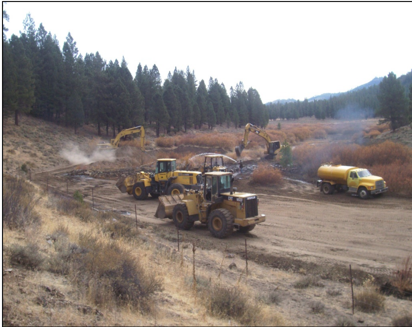
Work on the rock constriction plug. Rarely was all equipment in one photo frame.
