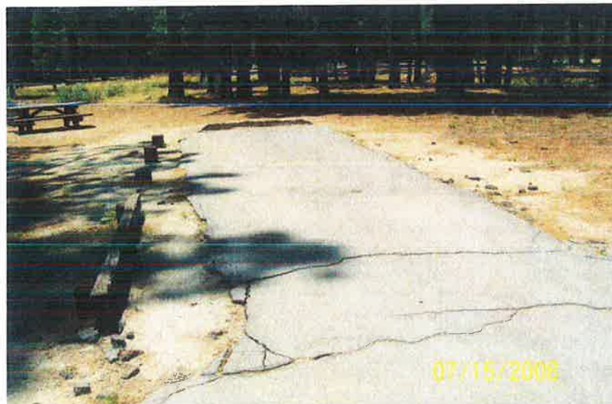
Figure 63. Example of deteriorated pavement typical in Lone Rock Campground
