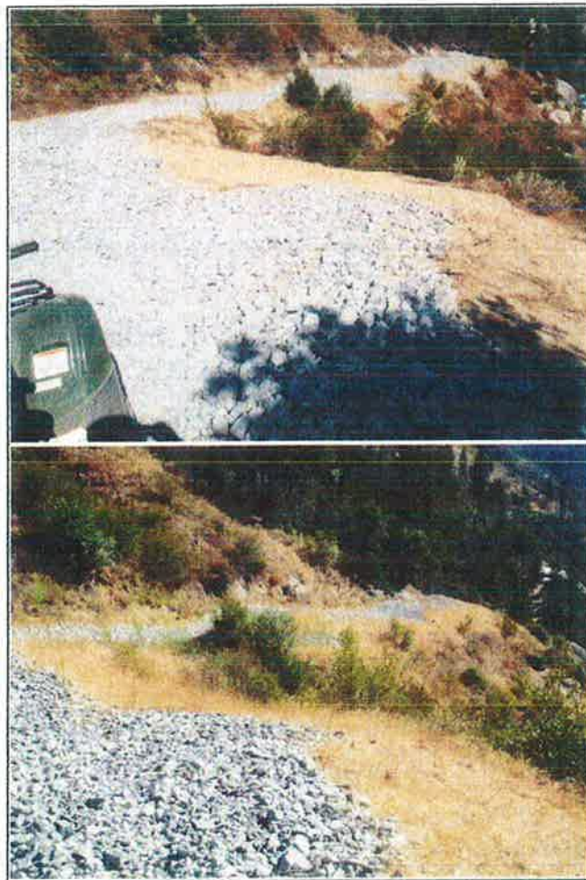
Figure 68. After OHV trail reconstruction, granitic soils are mulched and planted. In this Storrie Fire restoration project, native grasses persist 1.5 years after treatment.
