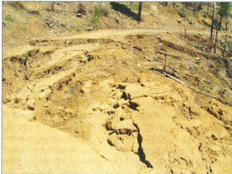
Figure 66. Road slump along NFS road 28N03 noted in BAER road monitoring (USDA 2009)
