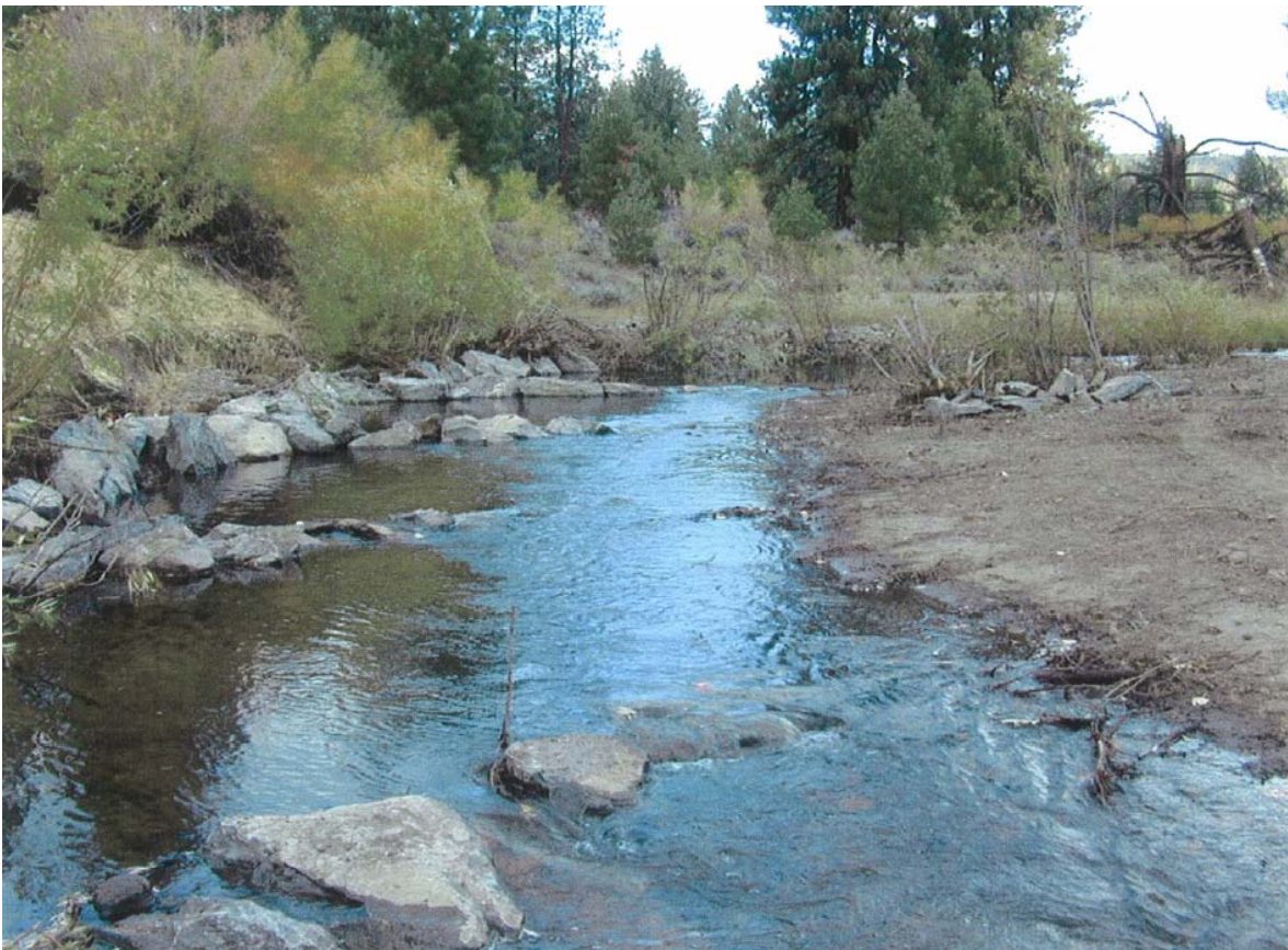
Little Last Chance Creek After Construction
