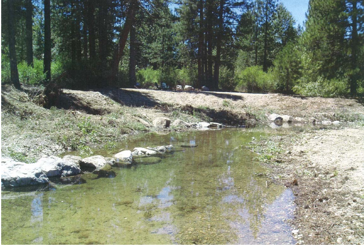
Boulder Vanes Constructed on Spanish Creek
